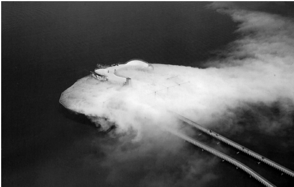
Figure 3: The Blur Building as (temporarily) constructed (Dimendberg, 2013, p. 154)
